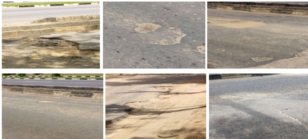
Fig. 2: Various failed sections of Edet Akpan Avenue
